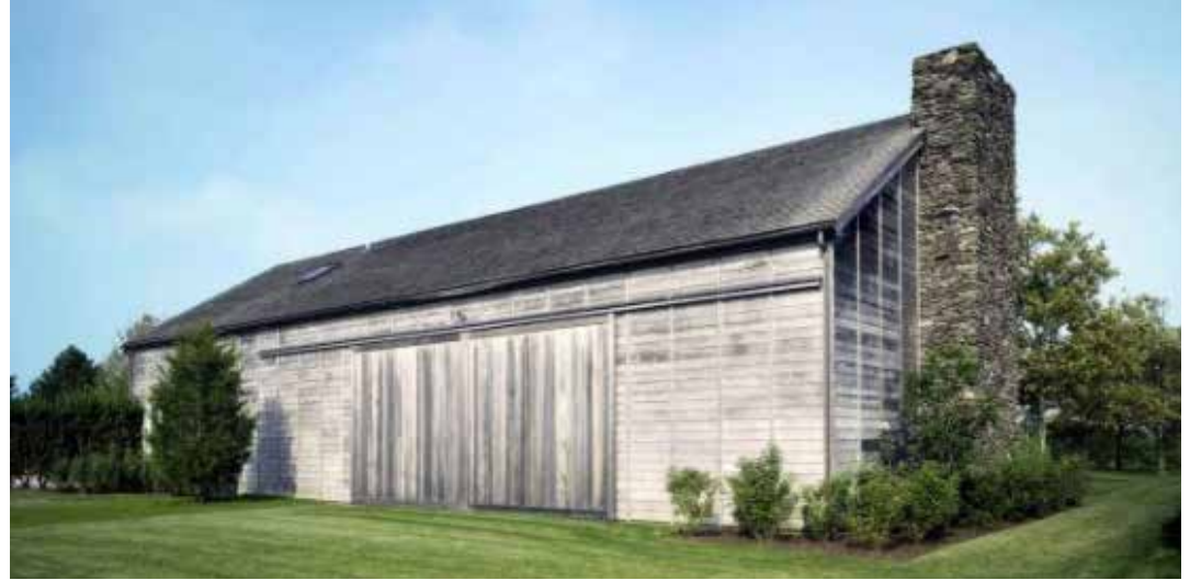
Sagaponack House, barn. Source: selldorf.com.
