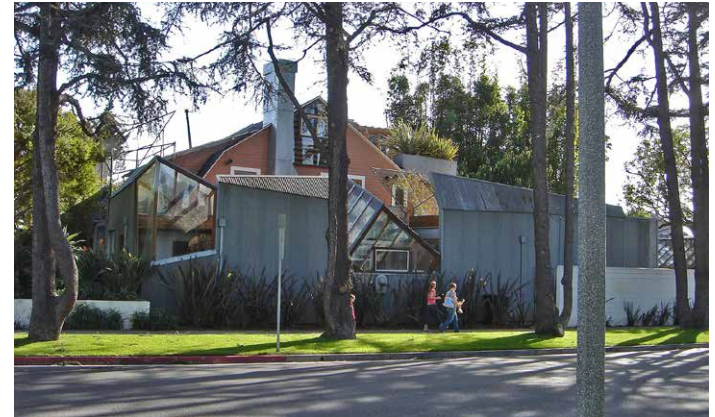
Gehry's former residence, side elevation. Source: archeyes.com.
