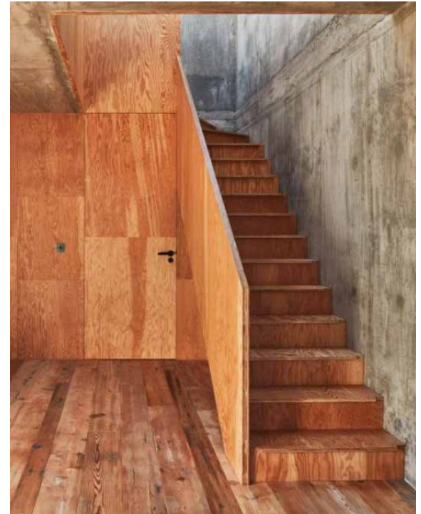
Mole House, stair detail. Source: wallpaper.com/ photo by Ed Reeve.
