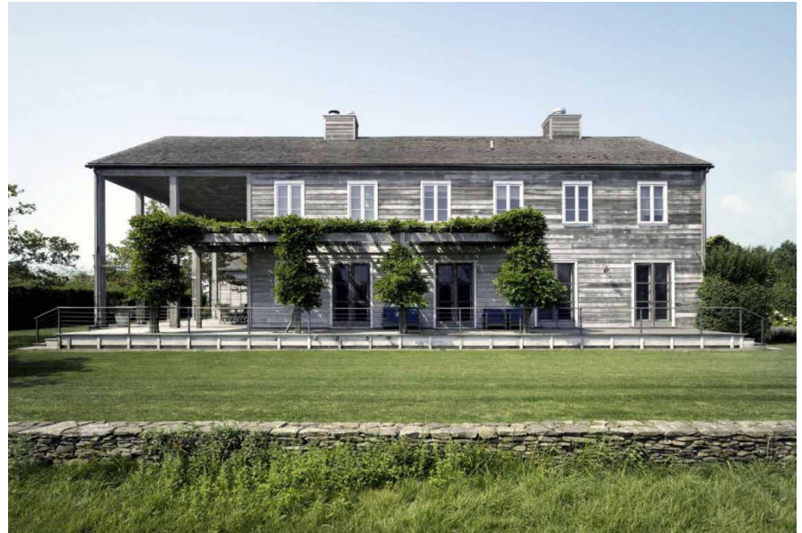
Sagaponack House & Studio, main elevation. Source: selldorf.com.
