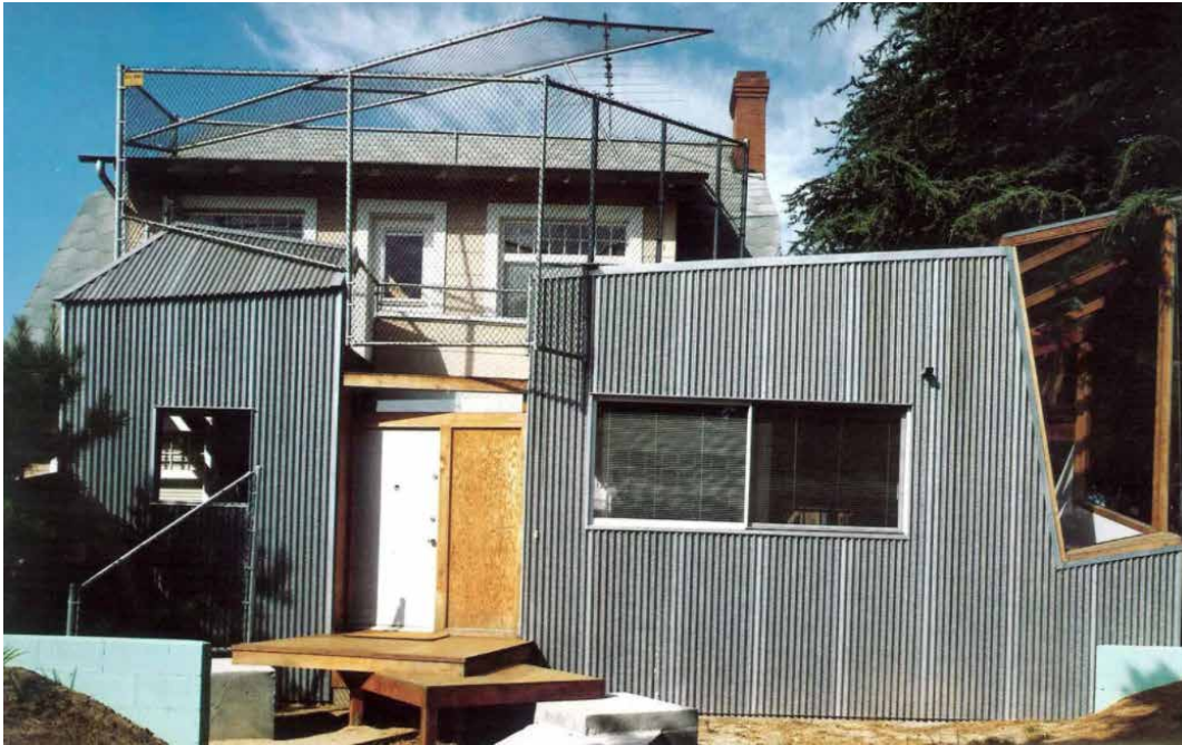
Gehry's former residence, front elevation. Source: archeyes.com.
