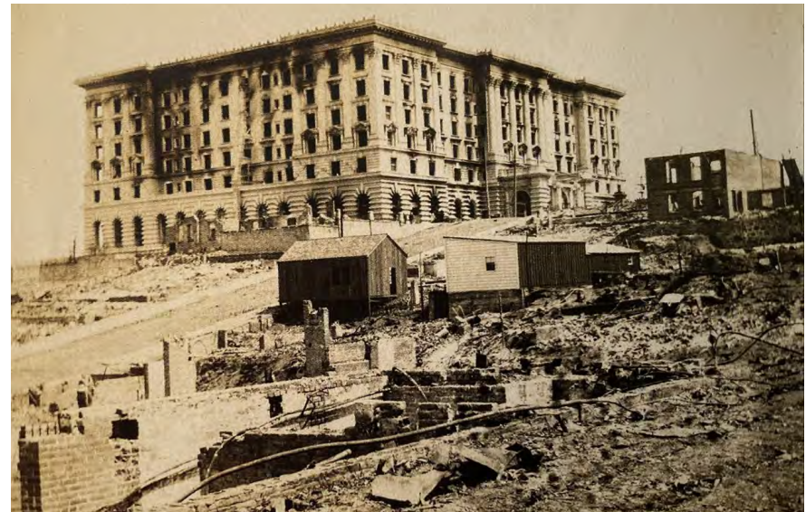
The Fairmont Hotel with interior gutted. Source: Kastner, op. cit.
