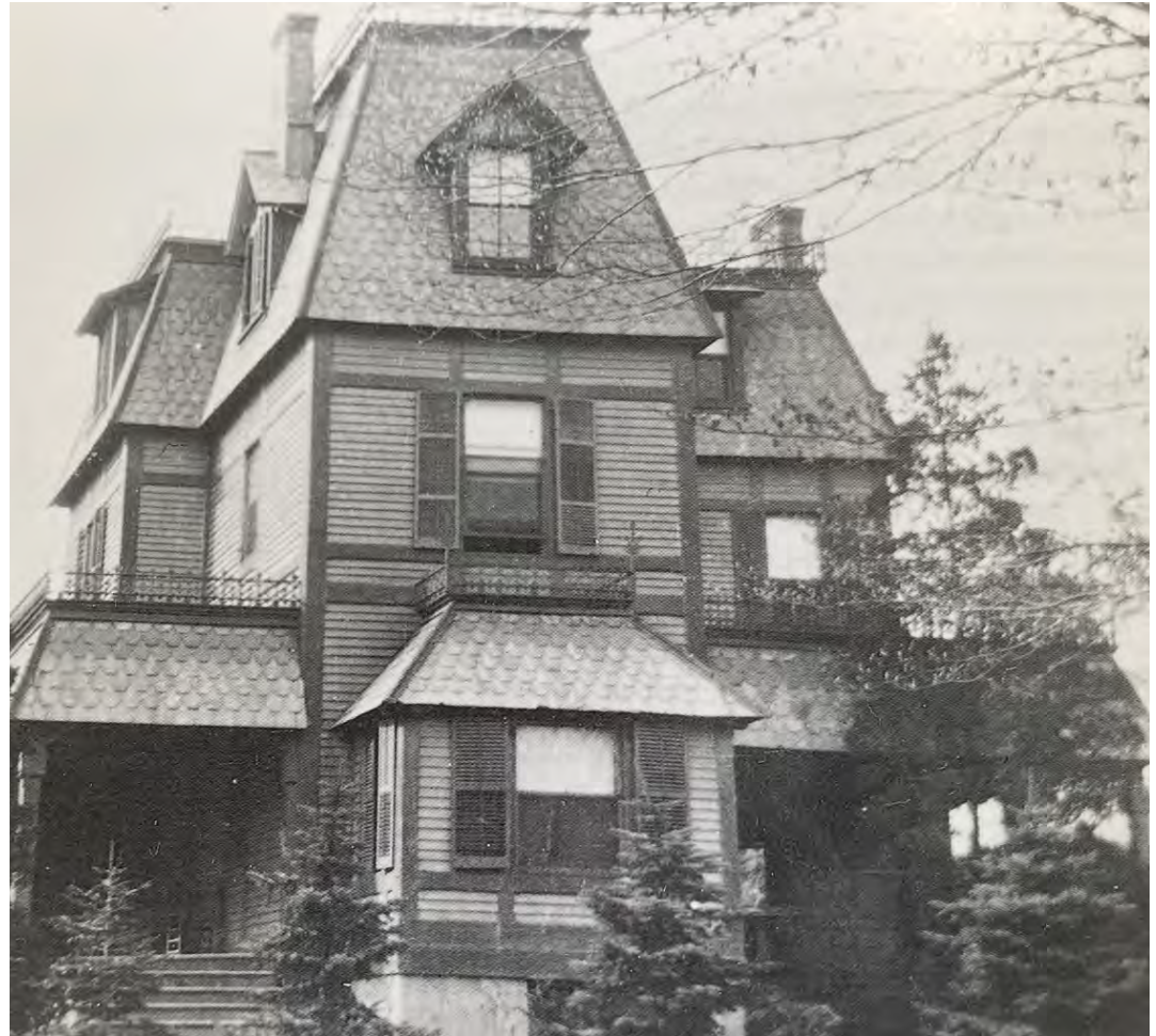
Richardson House, Staten Island, New York, 1869. Source: O’Gorman, op. cit.; Grace Church, Medford, Massachusetts, 1869. Source: Ibid.
